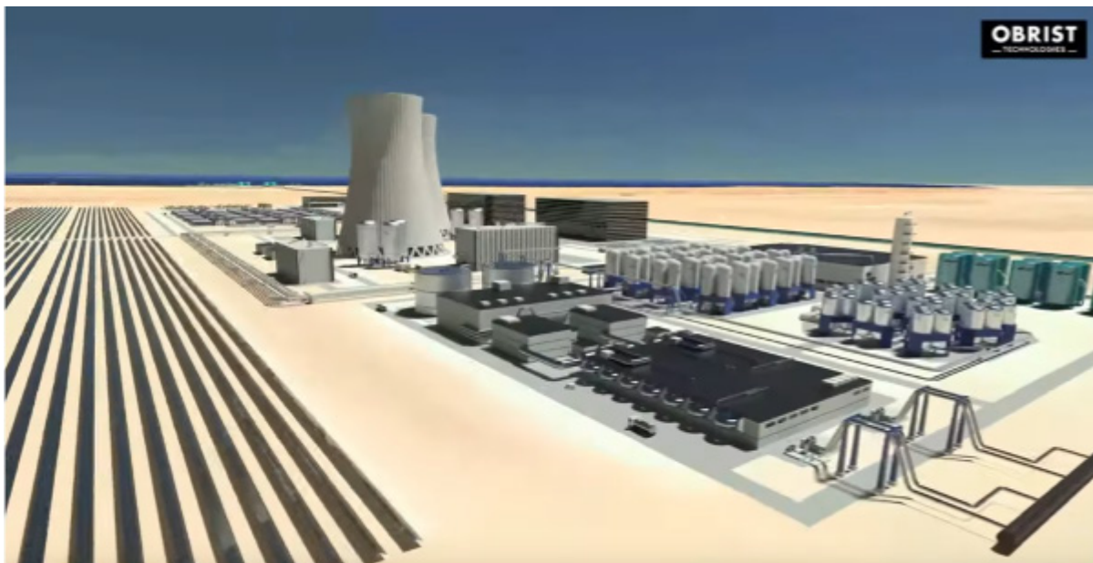
Figure 2: Model of a plant that uses solar energy to extract CO 2 from the atmosphere and to synthesize methane using hydrogen obtained electrolytically from desalinated seawater. Methane is the main raw material of the chemical industry as well as the starting material for other fuels and artificial biochar. Concept and design by Obrist AG .
